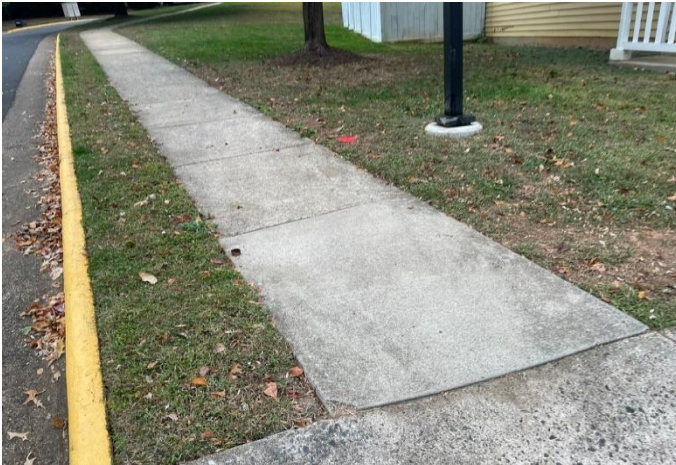
Concrete sidewalk overview
