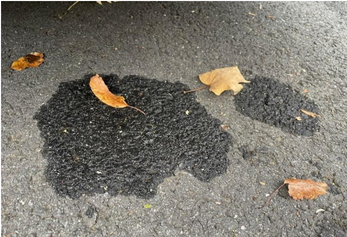
Chemical stains at asphalt
