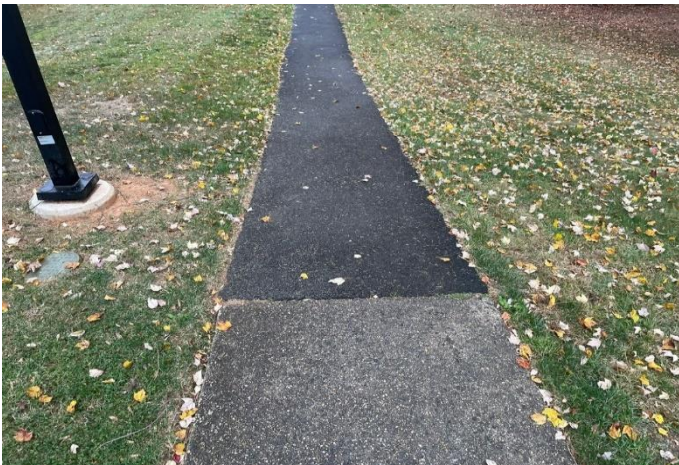
Old and new asphalt pavement
