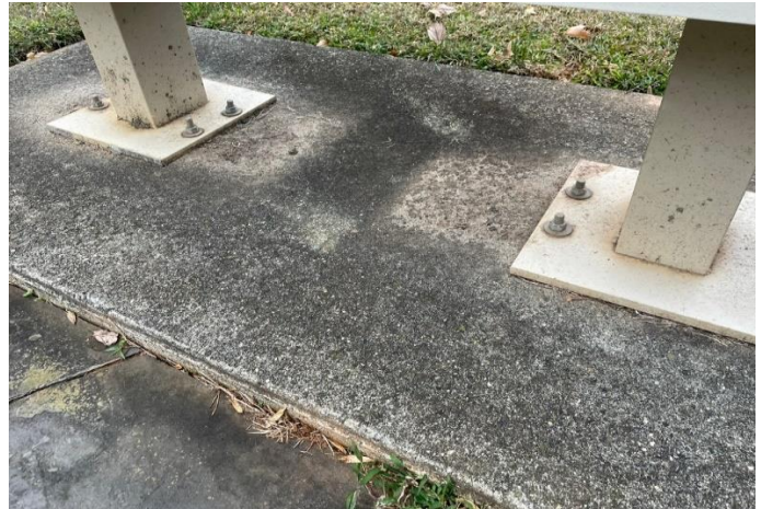
Concrete pad at mailbox stations
