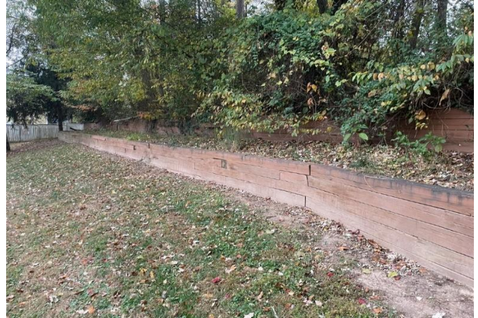
Timber retaining walls
