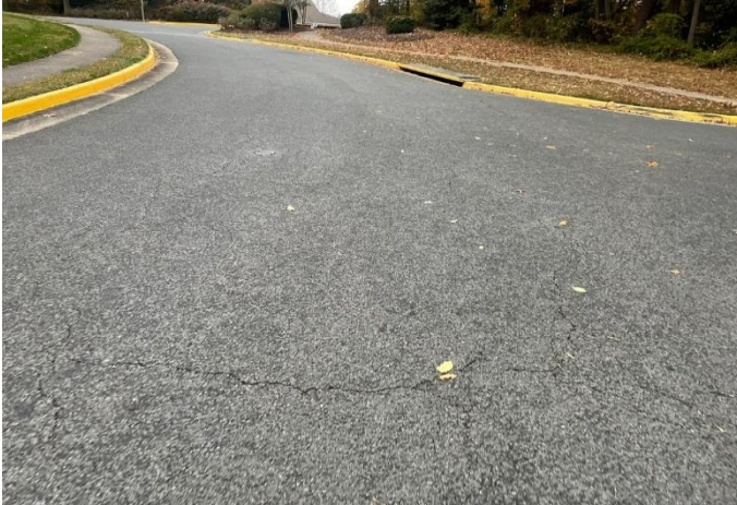
Asphalt street overview
