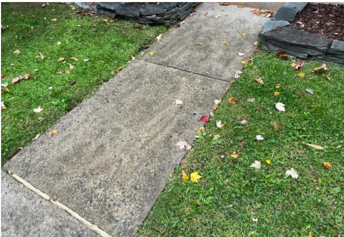
Concrete unit sidewalk
