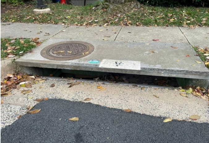
Catch basin overview
