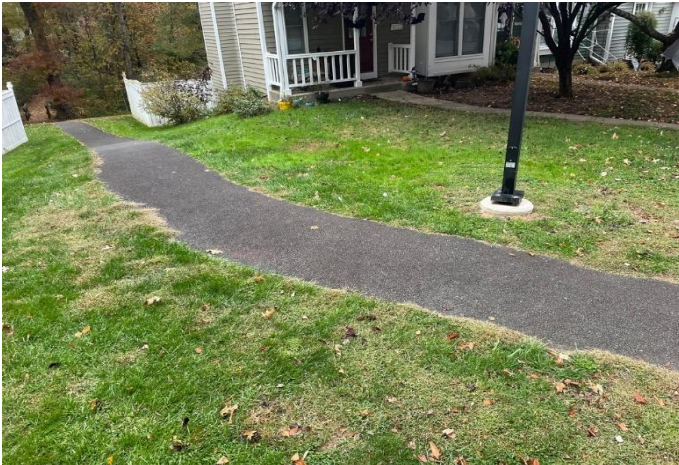
Asphalt path overview
