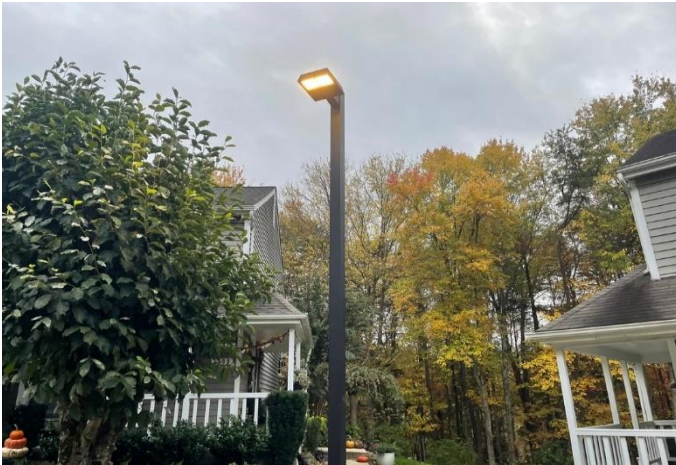
Light pole and fixture overview
