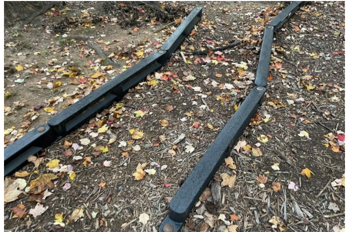
HDPE edging at playground area entrance
