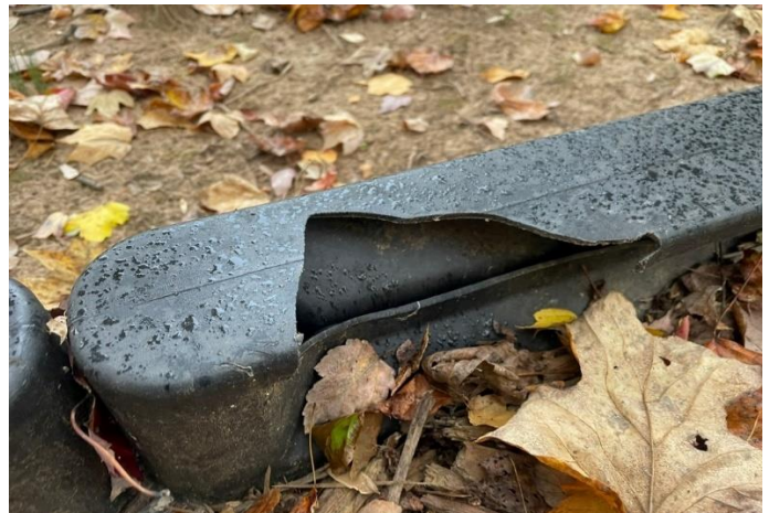
Damaged playground edging
