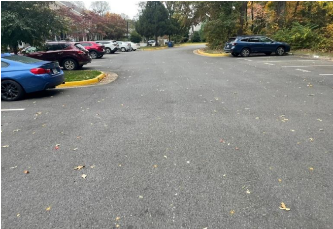
Asphalt pavement overview
