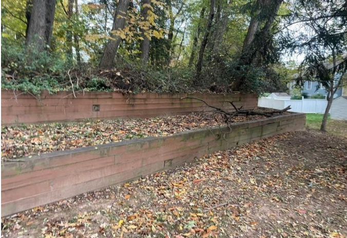
Timber retaining walls overview
