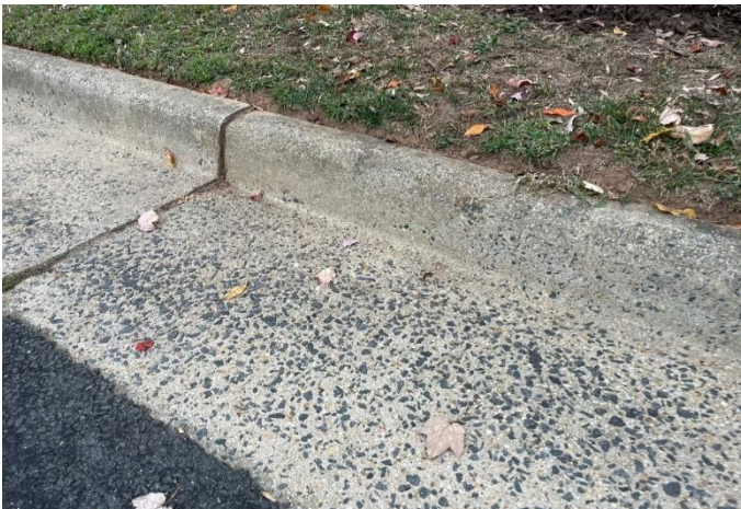
Typical concrete curb and gutter
