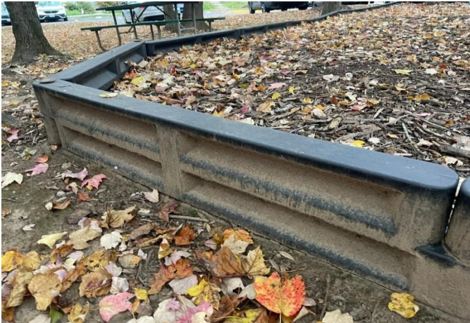
Playground edging overview
