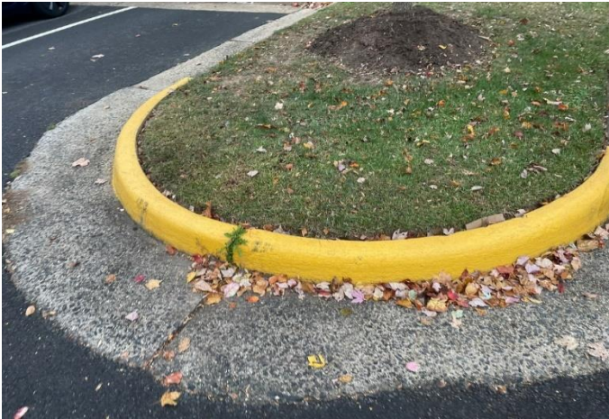
Concrete curb and gutters overview
