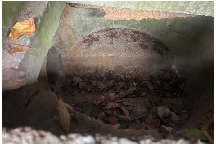
Typical catch basin interior
