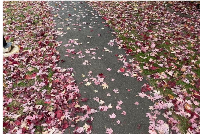
Asphalt path in good condition
