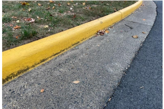
Painted concrete curb
