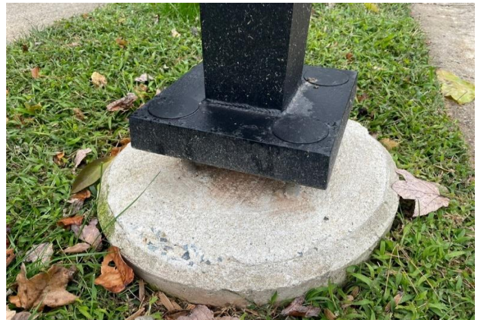
Concrete base at light pole
