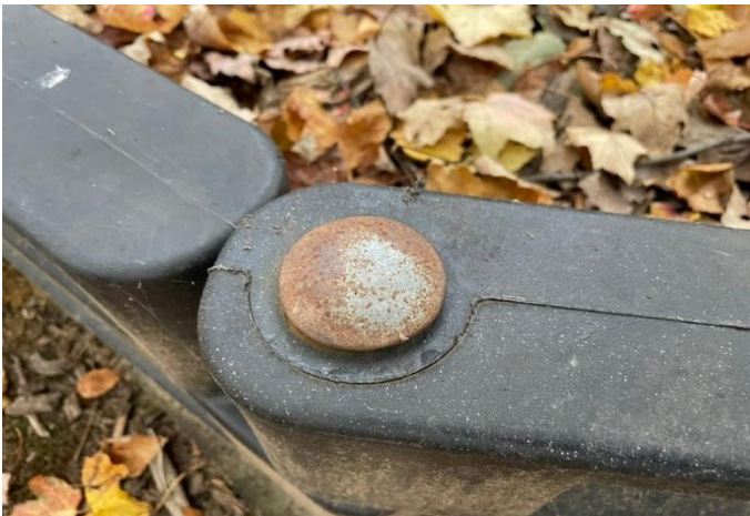
Rust at fastener
