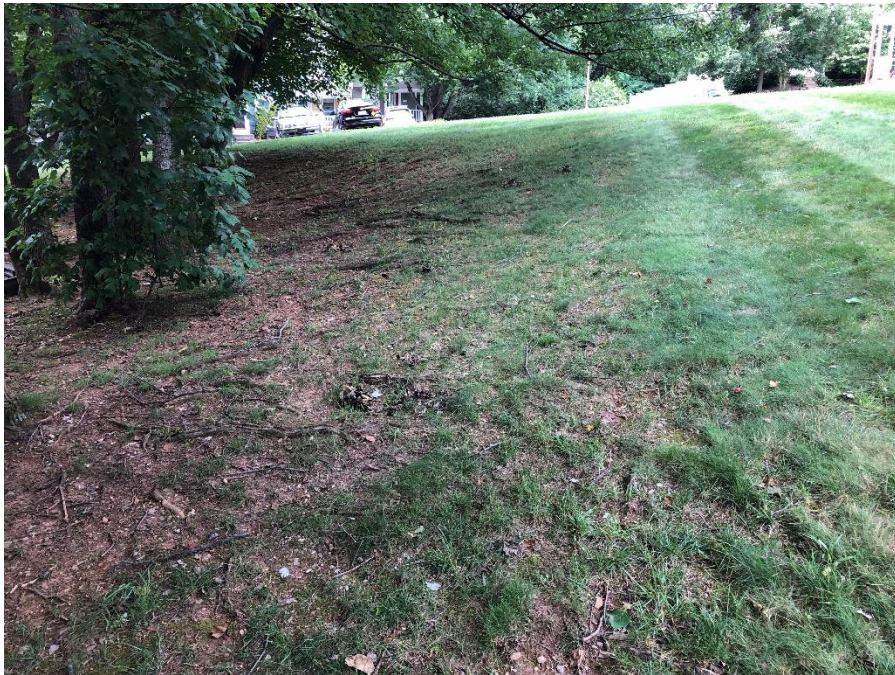
Photograph 16 – Steep-sloped area adjacent to tot-lot – note bare areas and exposed roots
