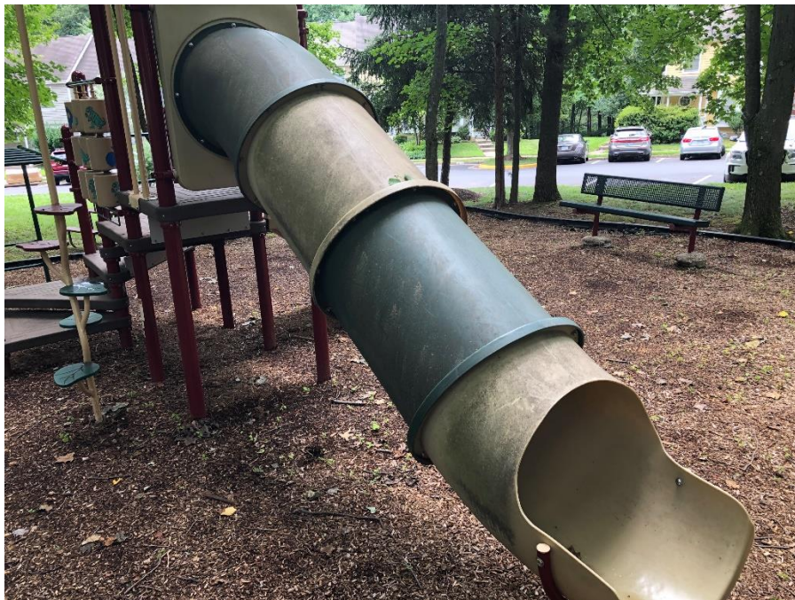
Photograph 8 – Pollution staining on slide
